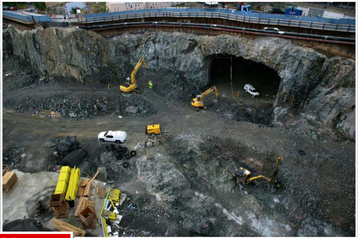
Liljeholmenstorget construction in June 2008
