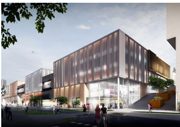
Largest Geothermal heating and cooling energy plant in Europe is being built beneath the shopping centre
