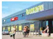
Åkermyntan Centrum, Stockholm Citycon's GLA 10,200 sq.m. Anchor tenants ICA, Lidl, health centre, library
