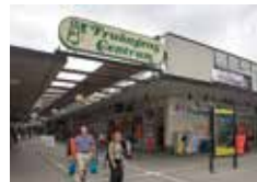
Fruängen Centrum, Stockholm Citycon's GLA 14,800 sq.m. Anchor tenants Coop, Systembolaget, Hemköp, Fitness24Seven, library, health centre
