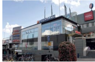
Forum Jyväskylä Citycon's gross leasable area 17,500 sq.m. Built in 1953/1972/1980. Extended and/or renovated in 1991.
